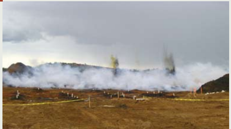
Blast densification of mine tailings
