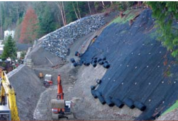
Debris flow mitigation
