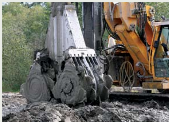
Advanced deep soil mixing techniques
