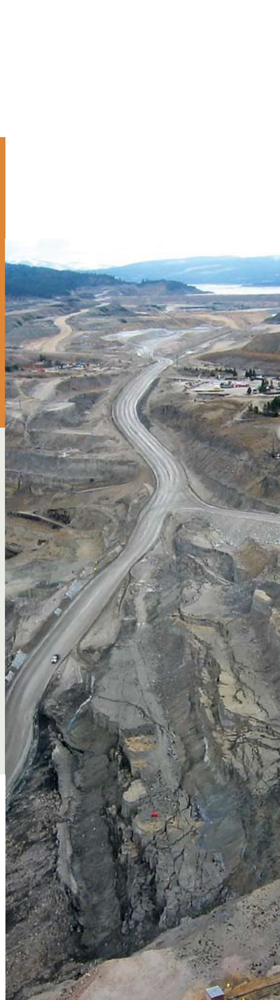
Slope depressurization for open pit extraction
